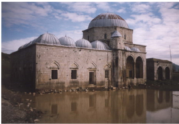
Fig. 2. The subsided and flooded Lead Mosque of Shkodra (18 th century)
